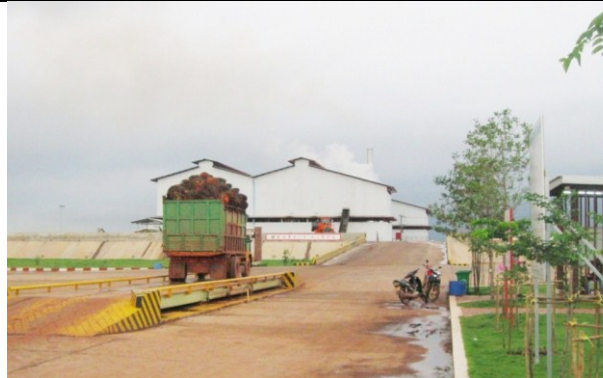
At new POM, weighbridge facility
